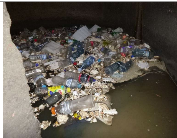
Sediment and trash build up in front of the weir and in pits generally – low capacity.
