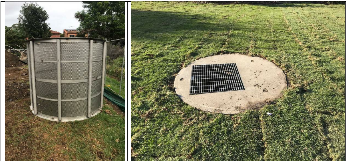
Replacement of GPT at Little Young Street, Cremorne.
