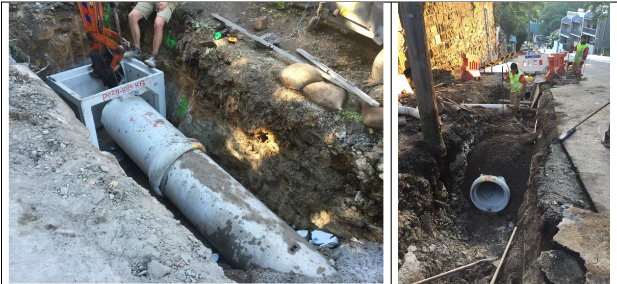
Pit and Pipe replacement at Bob Gordon Reserve, Lavender Bay.
