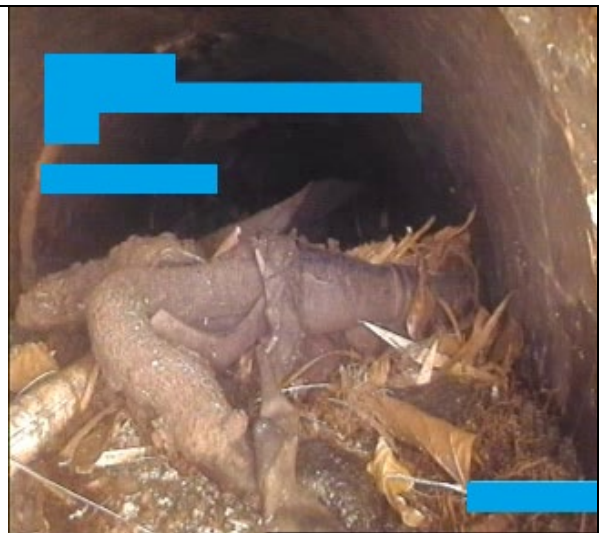
Stormwater Pipes in very poor condition – Tree root infiltrations and blocked
