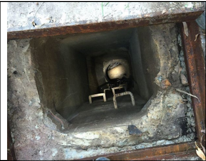
Sediment and trash build up in front of the weir and in pits generally – low capacity.
