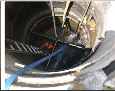
Sediment and trash build up in front of the weir and in pits generally – low capacity.
