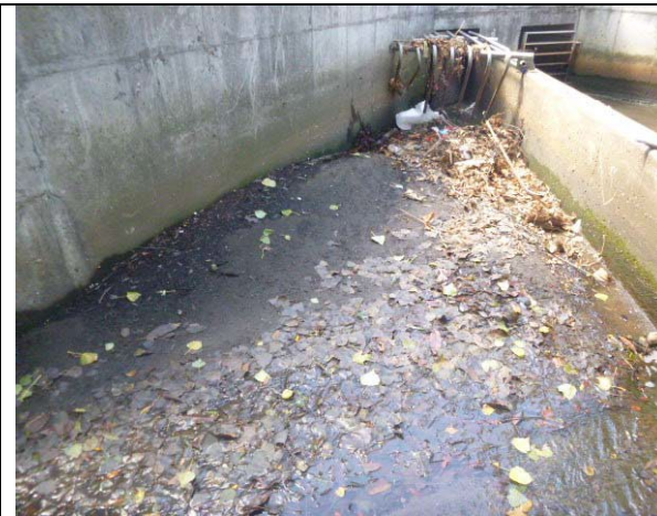
Sediment and trash build up in front of the weir and in pits generally – low capacity.
