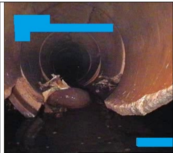
Stormwater Pipes in very poor condition – collapsed
