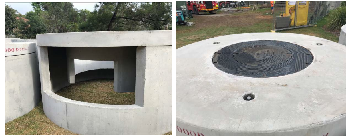
Replacement of GPT at Little Young Street, Cremorne.
