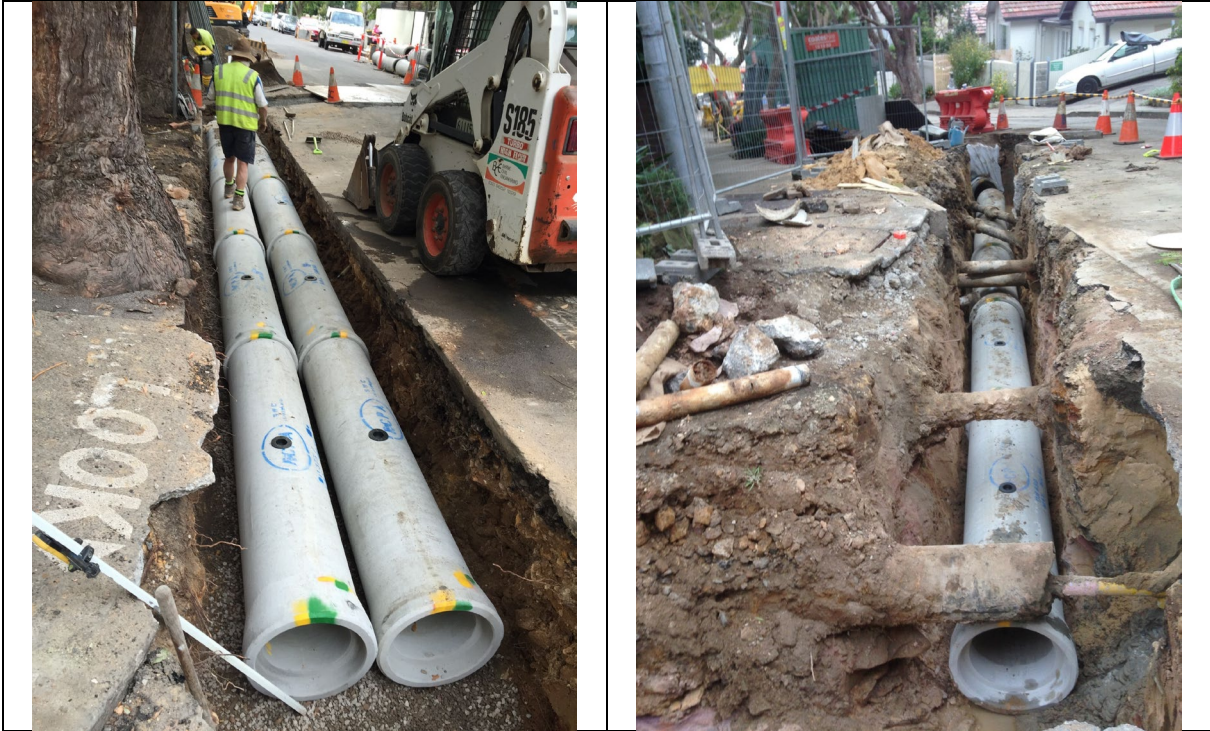
Pit and Pipe replacement at Carabella Street, Kirribilli.
