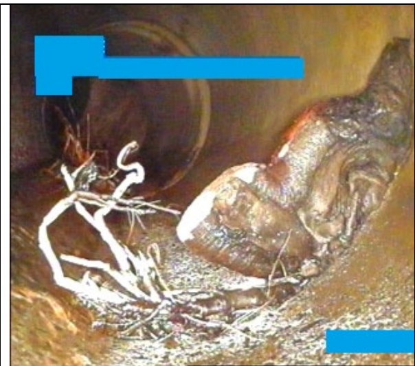
Stormwater Pipes in very poor condition – Tree root infiltrations and blocked
