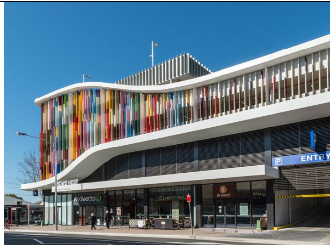
After - Alexander Street Car park Re-development- completed 2016 (Public Private Partnership) with Woolworths
