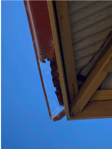
Examples of failed gutter and rotting timber in Property Assets in the North Sydney LGA
