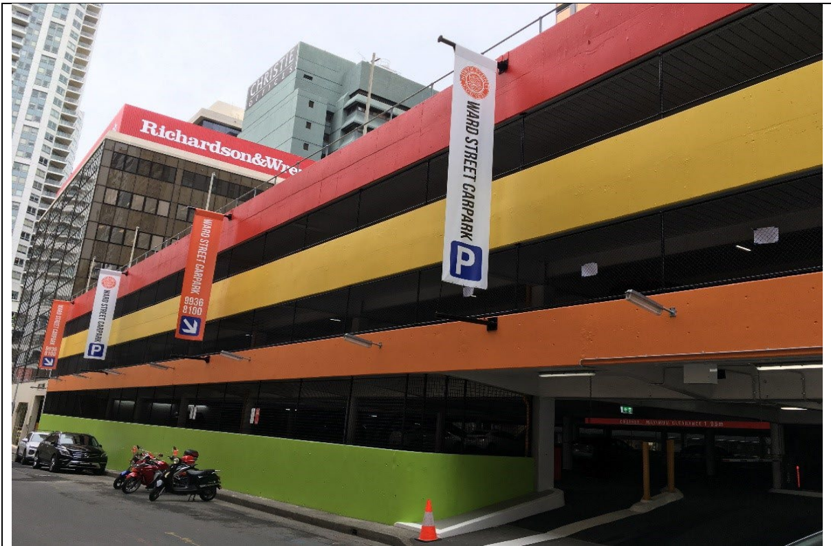
Ward Street Carpark – North Sydney Centre – Council took back possession of this three storey car park in the middle of North Sydney in August 2020 from Wilson Parking after the 50 year lease expired. The property in 2016 was valued at over $80 million on the open market in terms of development potential.
