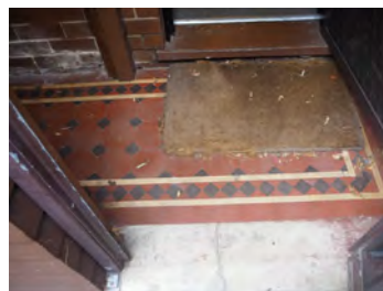
Figure 2. 66: Original encaustic tiles to verandah floor.
