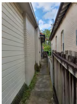
Figure 2. 112: View down west side passage.
