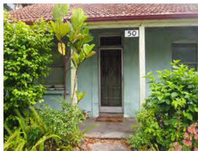
Figure 2. 2: No. 50 Parraween Street front door detail.
