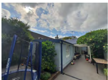
Figure 2. 18: Rear and east elevation of rear wing.
