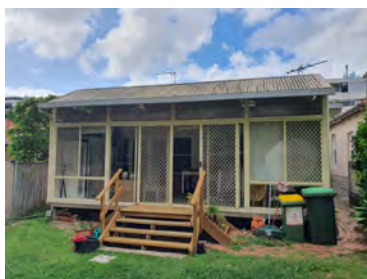
Figure 2. 111: Rear elevation of rear wing.
