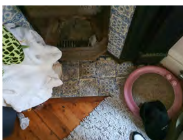
Figure 2. 134: Detail of tiling to living room fireplace.
