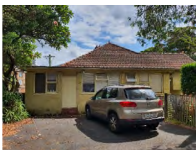
Figure 3. 35: South (side) elevation of No. 4 Macpherson Street.
