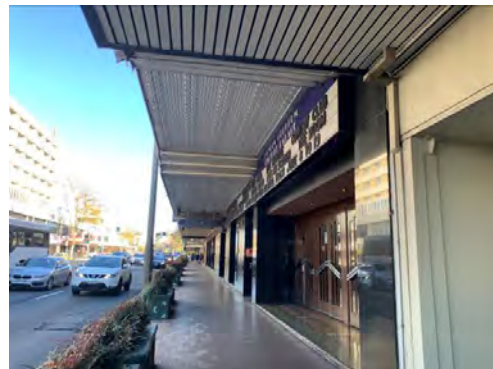
Figure 3. 64: Awning over original entry foyer, looking west.
