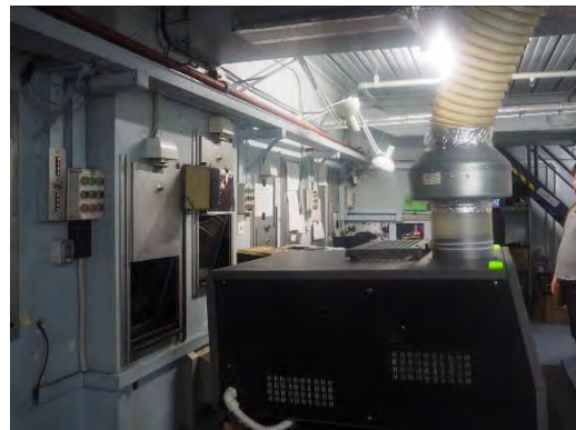
Figure 3. 80: Projection room to main auditorium
