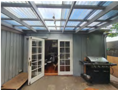
Figure 2. 51: Rear elevation of rear wing.
