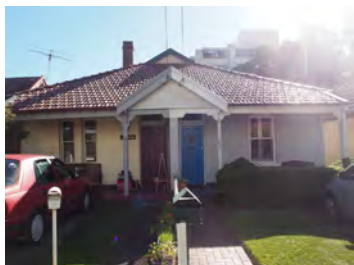
Figure 2. 76: Front elevation of Nos. 78 and 80 Parraween Street
