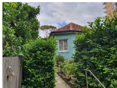
Figure 3. 21: No. 4 Prospect Avenue.
