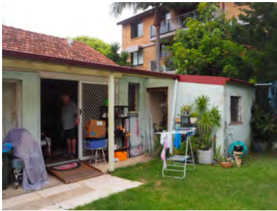
Figure 2. 7: Rear elevation with skillion addition.
