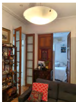
Figure 2. 155: Later French doors and enlarged door opening.
