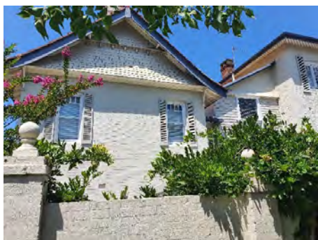
Figure 3. 54: Northern half of No. 23 Murdoch Street.
