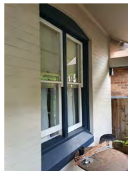
Figure 2. 110: Original windows to front elevation.
