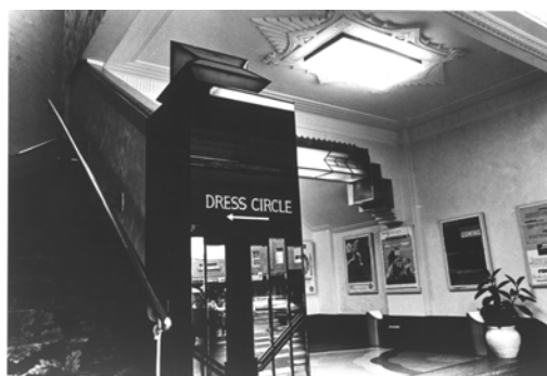
Figure 2. 35: Entrance foyer, c1960s. Source: Stanton Library
