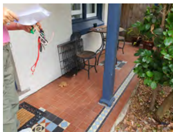
Figure 2. 109: Later tiling to verandah.
