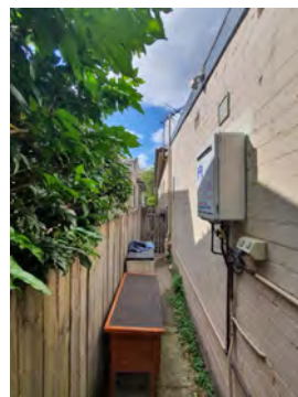
Figure 2. 94: Side passage to east side of house.
