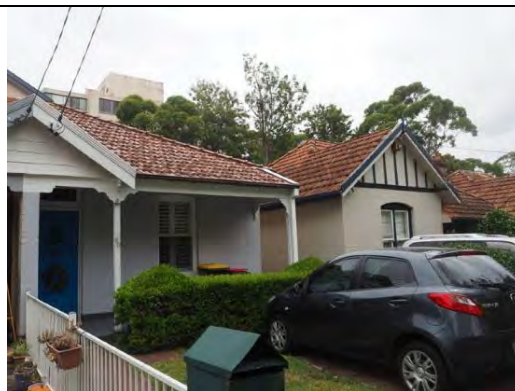
FIGURE 21: Frontage of 80 Parraween Street with No. 82 Parraween
