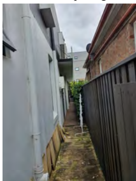
Figure 2. 46: Side passage showing east elevation.
