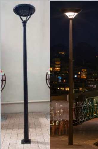
TYPICAL POST TOP LIGHT AS PER NORTH SYDNEY PUBLIC DOMAIN STYLE MANUAL AND DESIGN CODES
